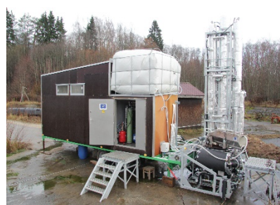
The biogas production facility - prototype
