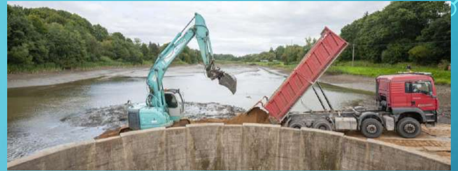
Temporary embankment formation for demolition works:
